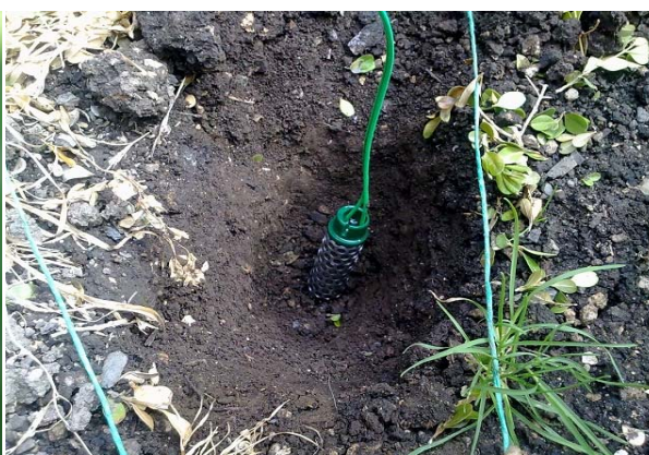
Fig 7. Installation of soil moisture sensor
